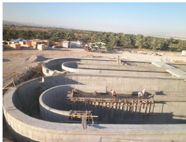
Figure 25: JWWTP under construction, 2013
